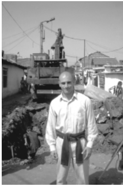
Stephen Kooshak '98 overseeing work site providing water and sewage lines
