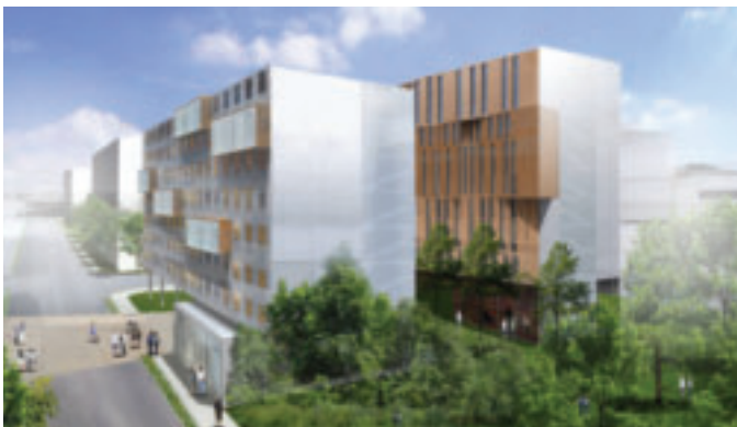
Computer generated image of dormitory building / Ile Seguin 2010
